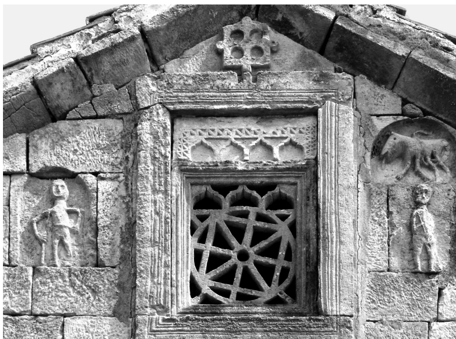
Fig. 5. St. Nicholas Church at Žegljane, western facade (photo courtesy of Slavica Krstić)
