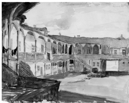
Fig. 18. The inn "Manuc Han" in Bucharest. View from the courtyard
